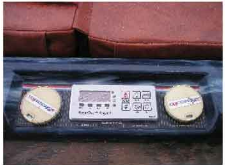
Final view of installed digital keypad.
